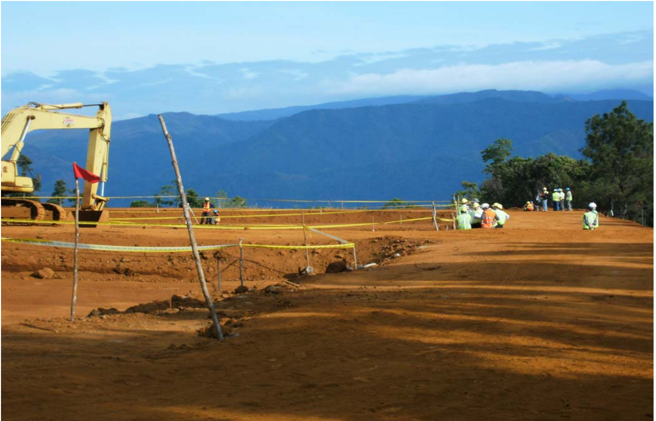
Trial heap leach pads under construction at Acoje
