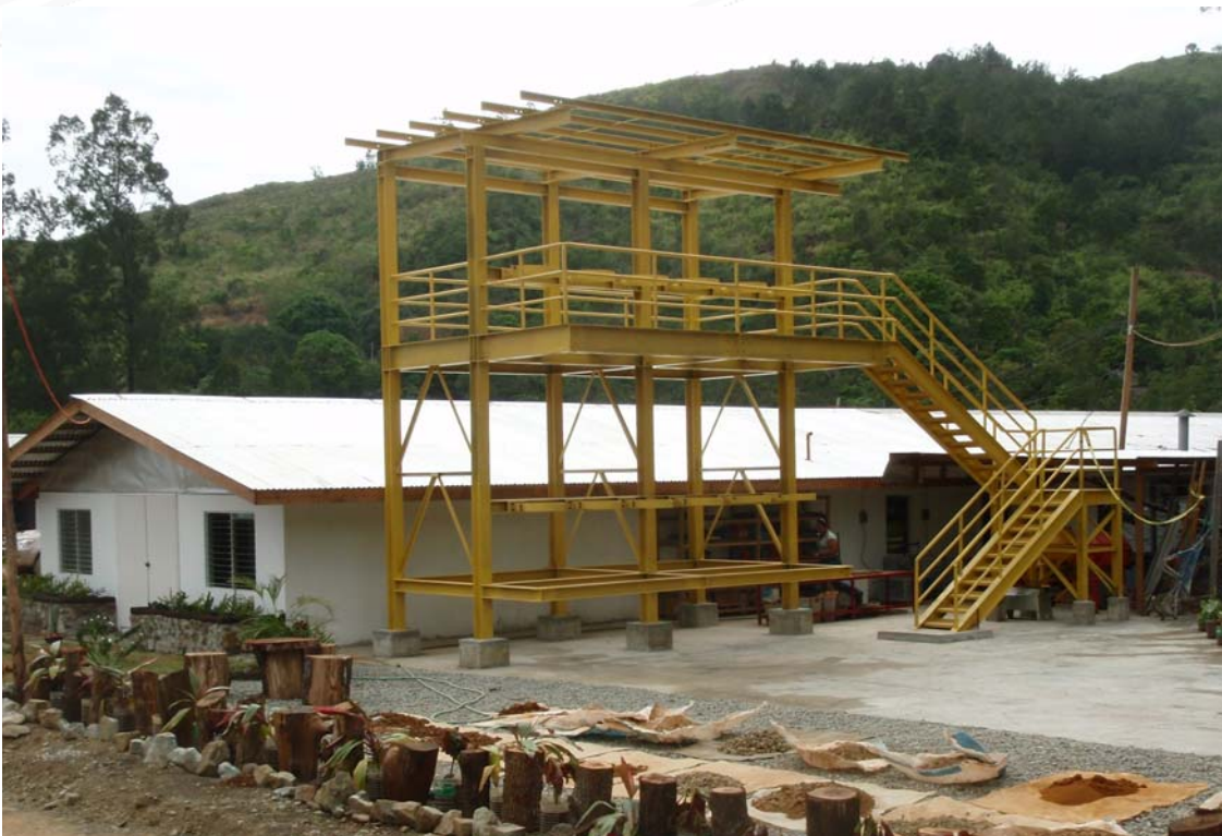
Fig 2 Acoje Research Lab. Steel works for 4m columns complete.
