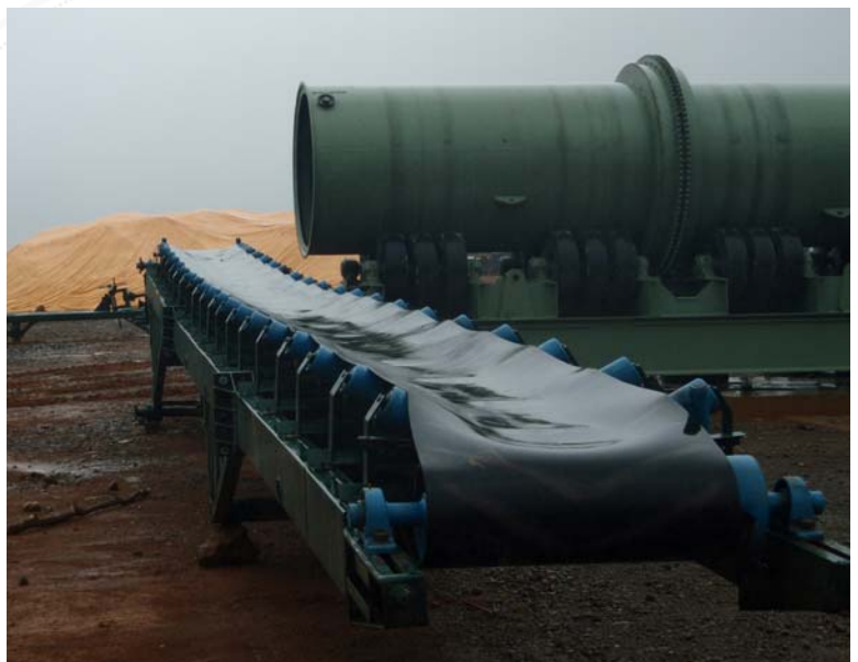
Fig 1: Agglomerator and stockpiled ore ready for heap leach trial
