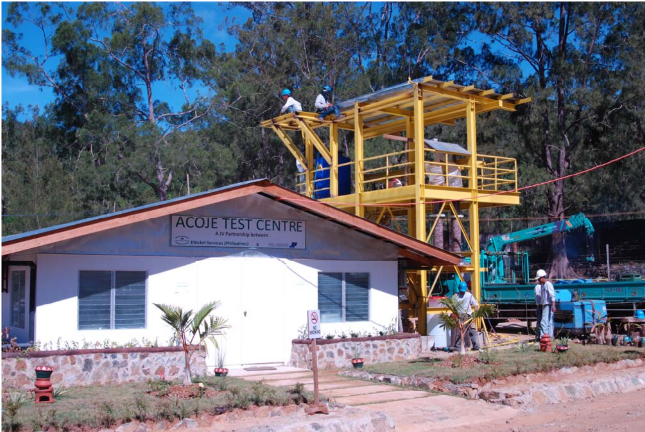
Fig 2: Acoje Test Centre. 4m test columns being installed at rear.
