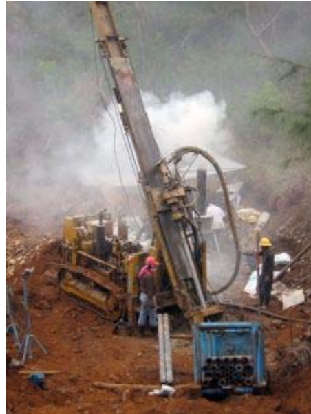
Drilling at Central Block
